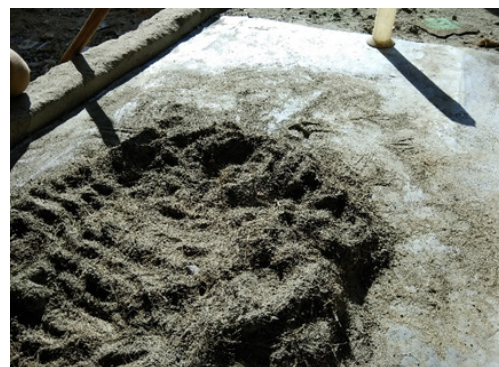
Figure 5. Mixing of fibre in concrete
