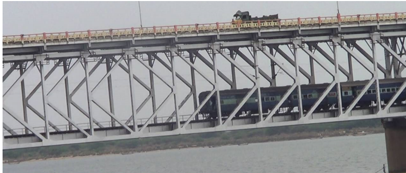
Figure 1.1: The Godavari Bridge, Rajahmundry, Andhra Pradesh, India.
