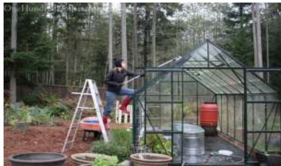
Fig.1. Greenhouse Roof Cleaning Manually Using Brushes
